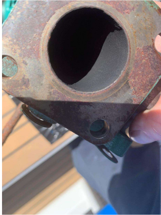
Turbo Exhaust inside Chamber Before the Turbine1. No Soot Accumulation there.
