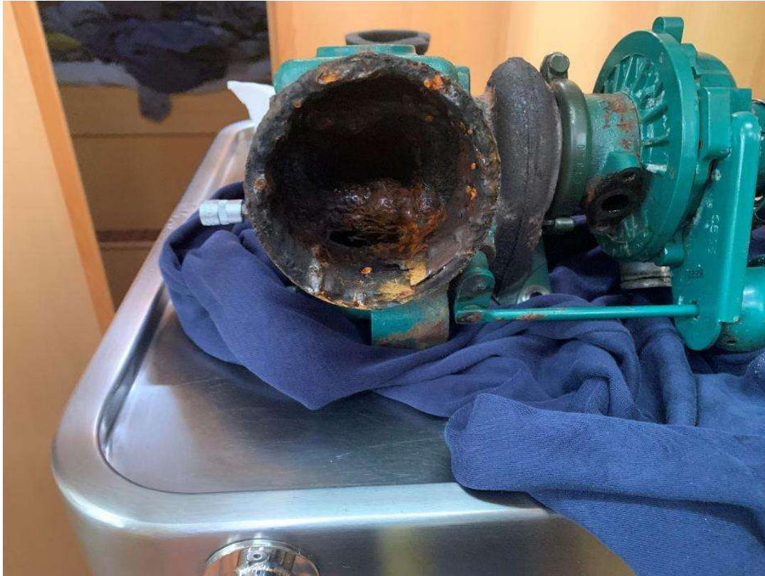
Severely Corroded Exhaust Elbow After Water Injection.
